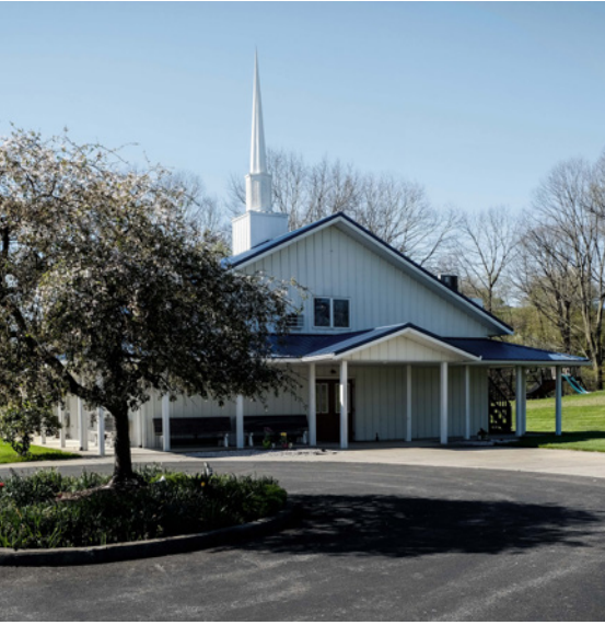
The chapel from the parking lot
